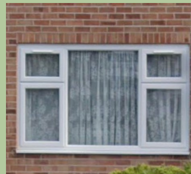
Typical white UPVC window with brick window head, common throughout the area.
