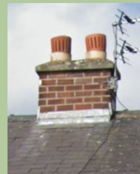
Brick chimney on slate roof typical to the Poplars Avenue area.
