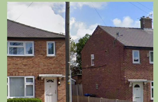
Gabled and shallow-hipped roofs are both used throughout the area in irregular patterns.
